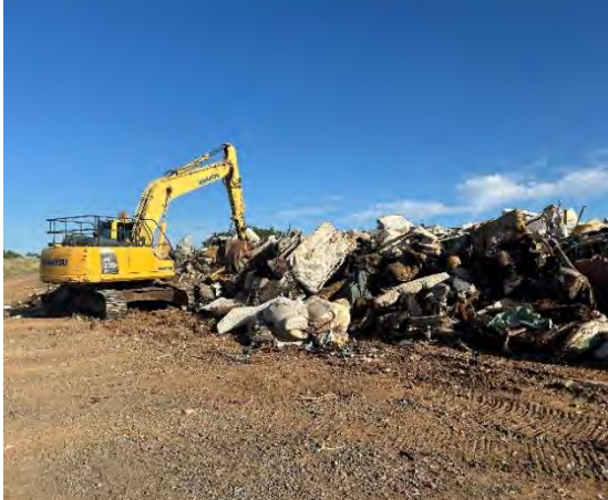
Mattress Cleanup underway
